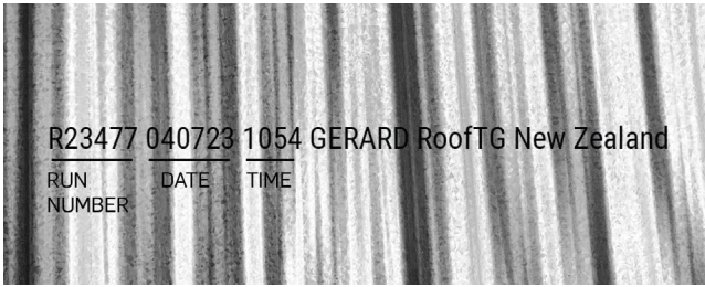
Figure 2.4.2 Label on the back of the tile
