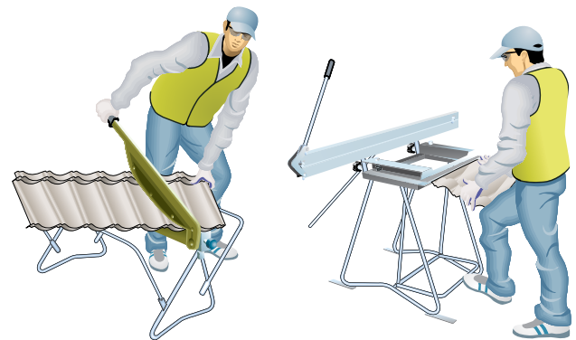
Figure 14.7.7.2 Valley tile being cut then bent
