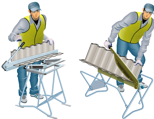
Figure 6.2.6.3 Ridge tile being bent then cut
