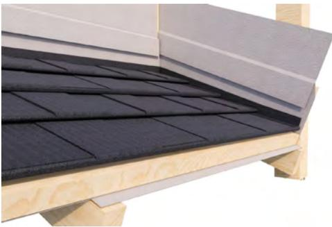
Fix the side flashing to the support nog in the wall. Wall underlay should lay over the top of the side flashing, while the roofing underlay should lie between the side flashing and the wall.
