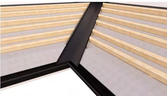
Using a nail or valley clip, secure the valley tray into place. If using nails, ensure you do not penetrate the valley by bending nails over the rail, rather than screwing through the valley tray.
