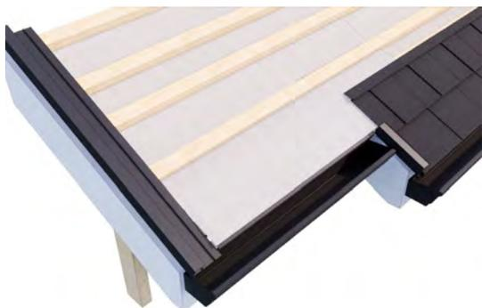
Measure and cut the head off the first course of panels at the short edge of the roof. The head should align with the head of the already-installed panels. Hook the nose over the eaves flashing and fasten in place.
