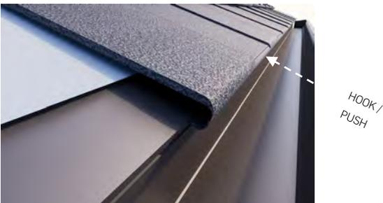
Secure the panel with five fasteners evenly spaced at the head of the panel.
