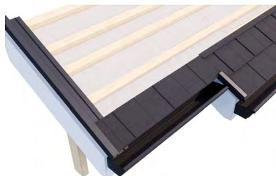
Fasten the shortcourse flashing in place, in alignment with the head check of the already-installed panels.
