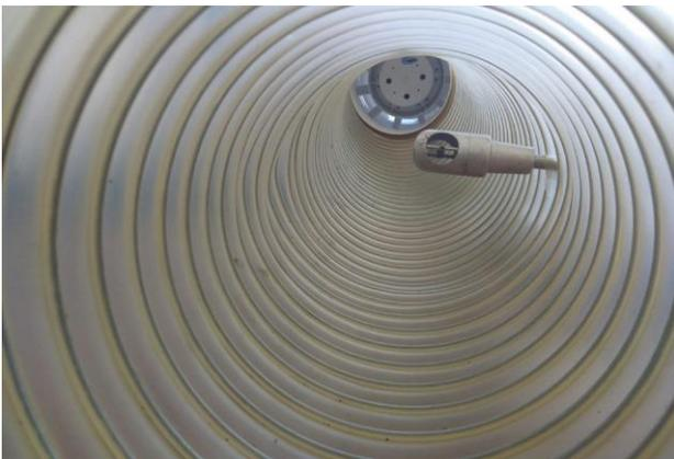
Anemometer in duct
